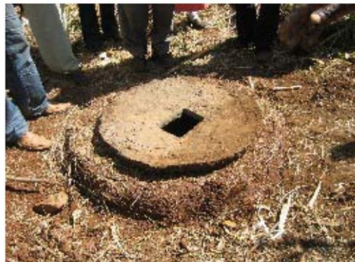
*The slab is then moved on to the ring beam so it is supported equally all round. It is bedded in so the slab is well supported all round. Extra mortar is made and placed around the slab.*
