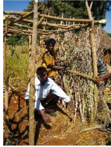
*The four corner posts are placed in holes around the slab and ring beam. Smaller poles are placed over the roof and on the side walls of the structure. Suitable traditional walling and roofing material is found and added to the structure.*
