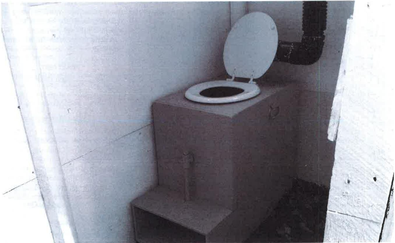
The CRAPPER. The handle in front is used for rotating the drum, and the waste is removed at the side.
