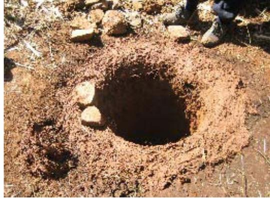
*The mix of mud and grass is made up and laid around the rim of the pit. Then flat stones are found and laid around the pit. These can extend for up to 30cm around the pit. The stones are bound by the soil. The reinforced soil is smoothed off ready to add the slab.*
