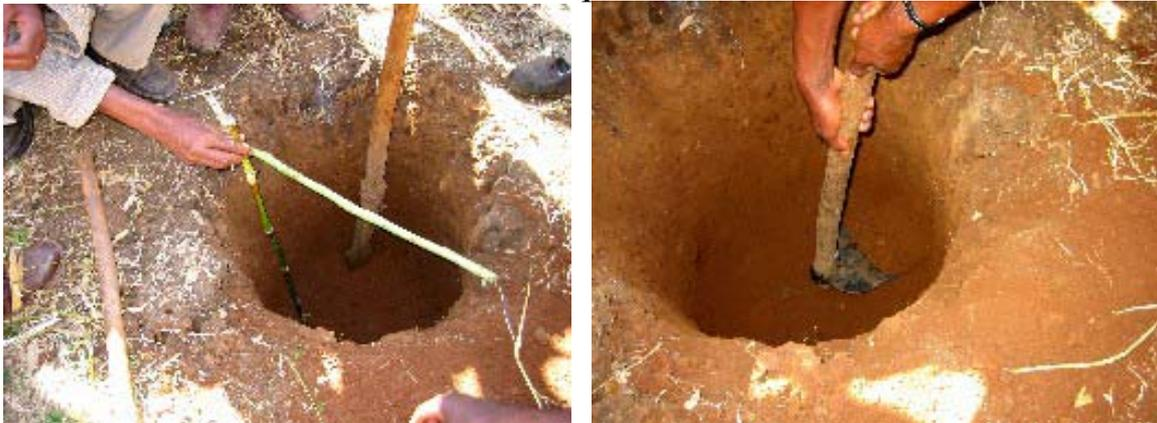
*The larger the diameter of the hole and the deeper the pit, the longer the pit will last. Some people may prefer smaller holes if they want to plant more trees, but this means moving the slab and “toilet house” more often. The larger the pit is, the longer it will take to fill up and moving the slab and house does not need to take place so often.*
